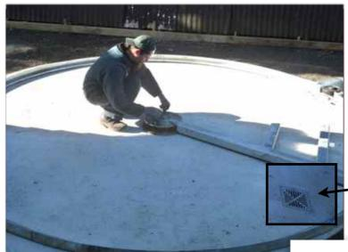
The turntable is constructed on a level, reinforced concrete pad 4.3 metres in diameter and 150mm thick. The pad needs to be 100mm below the desired finished driveway level.
